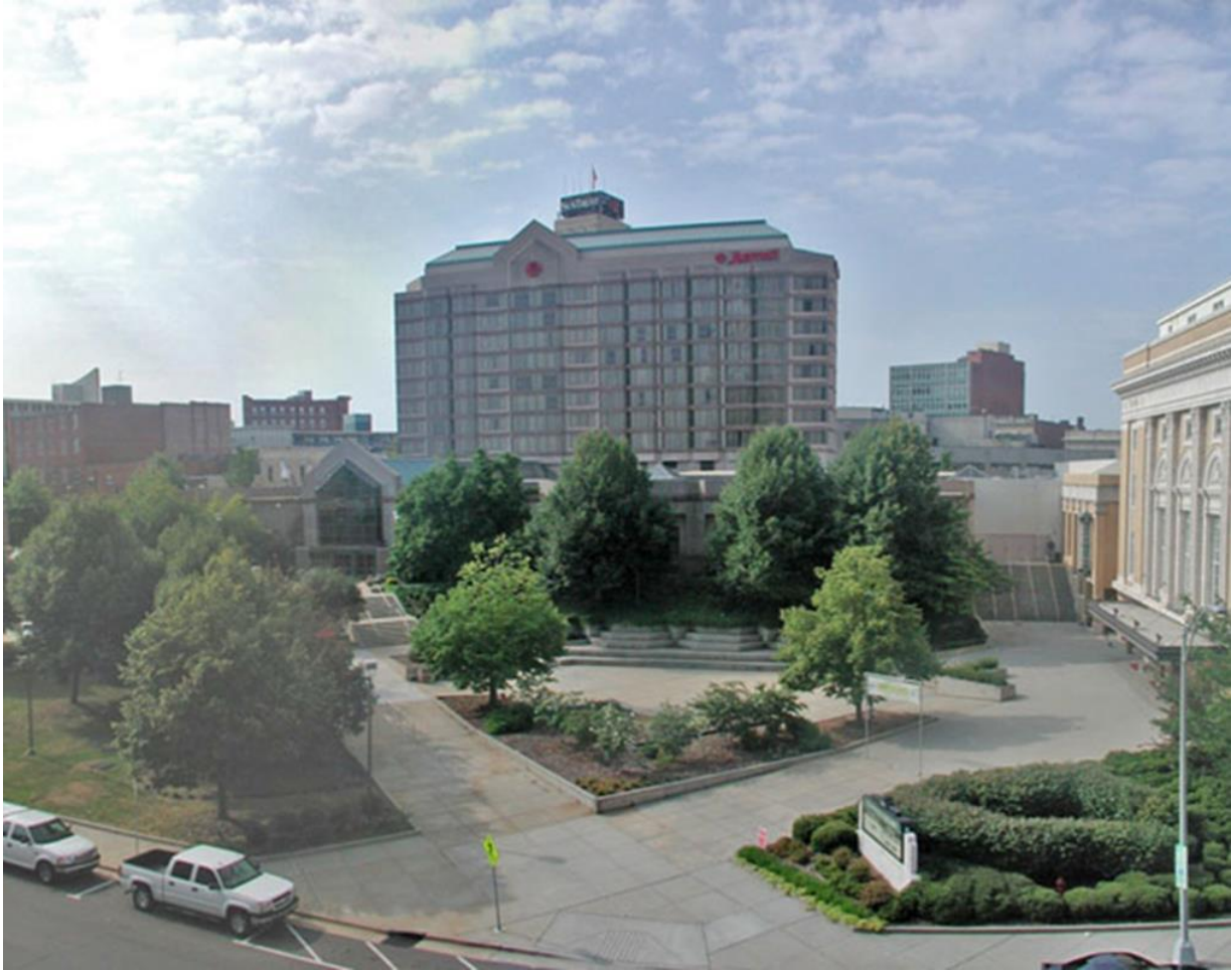
Convention Center/Carolina Theatre Plaza - Existing Condition
